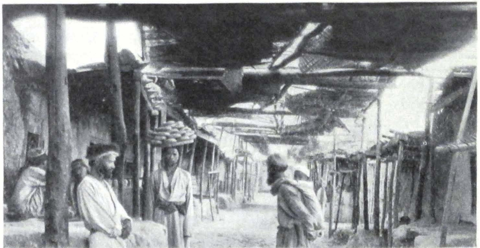
1. THE MYSTERY PLAY AT HEMIS : A CROWD OF LADAKHI MEN AND WOMEN WATCHING THE PLAY FROM THE BALCONY OF THE INNER COURTYARD IN HEMIS MONASTERY. 2. THE MAIN BAZAAR STREET OF KHOTAN: THE MAIN STREET WITH MUD-BUILT HOUSES ON EITHER SIDE IS COVERED WITH AN AWNING OF STRAW MATS.
